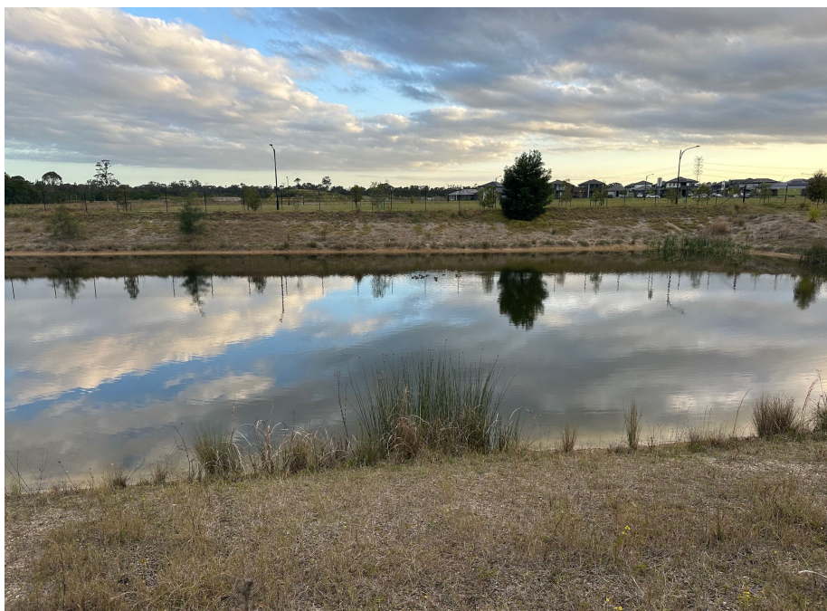
Figure 3 The OSD basin on the proposal site. Taken facing south.
